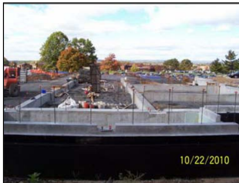
Figure 2: Grade Beams & Foundation Walls at East Side of Building
